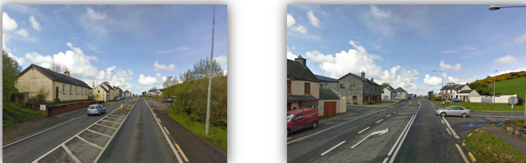
Plate 3-1: Existing N4 through Castlebaldwin
